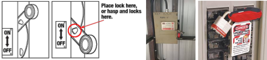
Figure 1: Electrical lockout.
