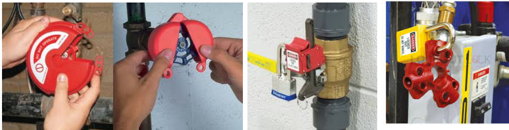
Figure 2: Hydraulic and pneumatic lockout.
